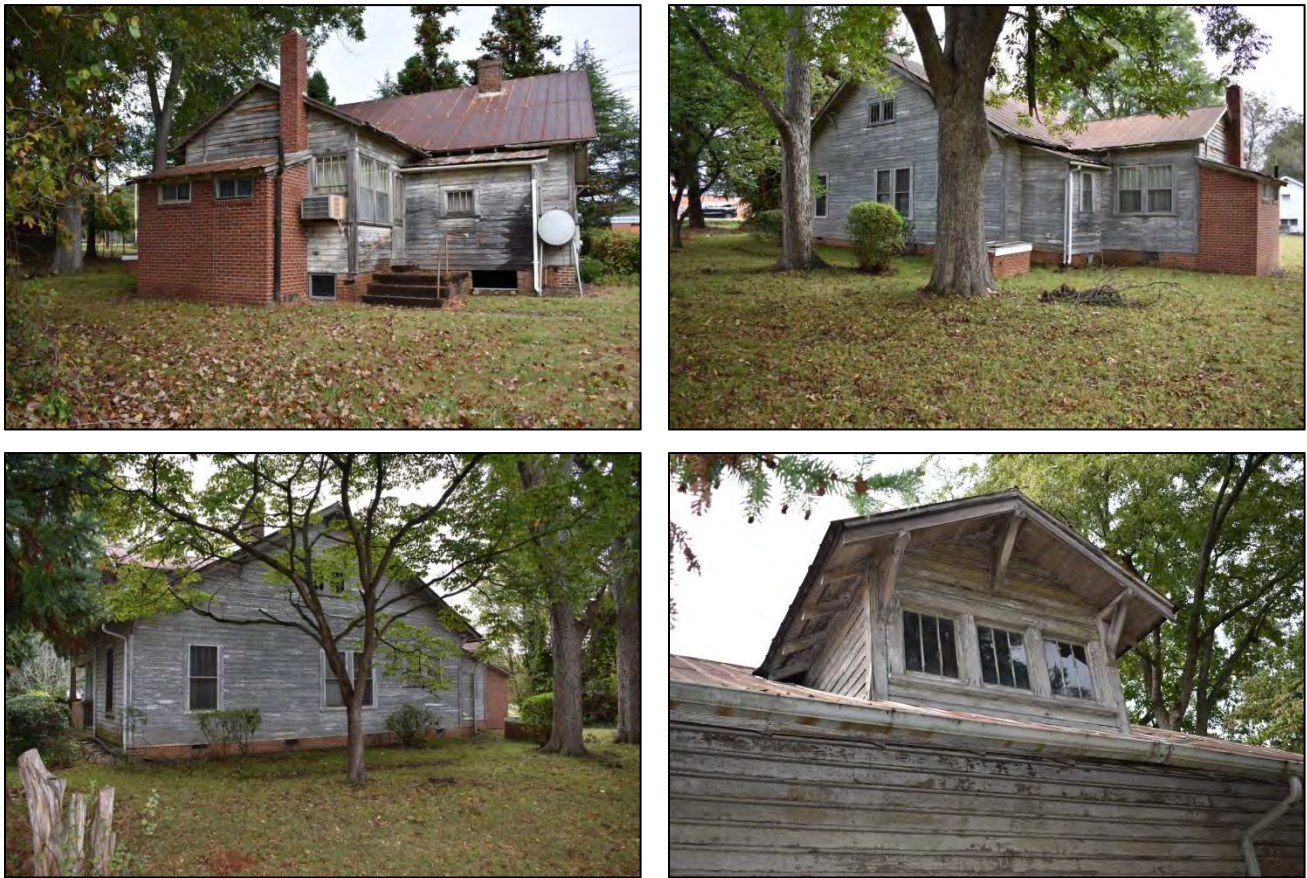
Figure 5: Left, rear (southeast) elevation; right, southwest corner; bottom left, side (western) elevation; bottom right, detail view of dormer found on primary elevation.
