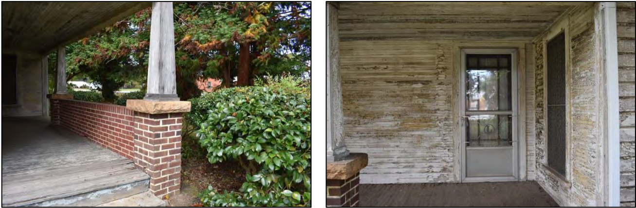
Figure 6: Details of the front porch.
