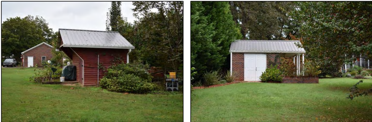
Figure 24: Left, side (eastern) elevation west shed; right, side (western) elevation of east shed.
