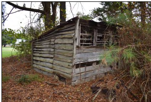
Figure 12: View of the front (southern) elevation of the chicken coop.
