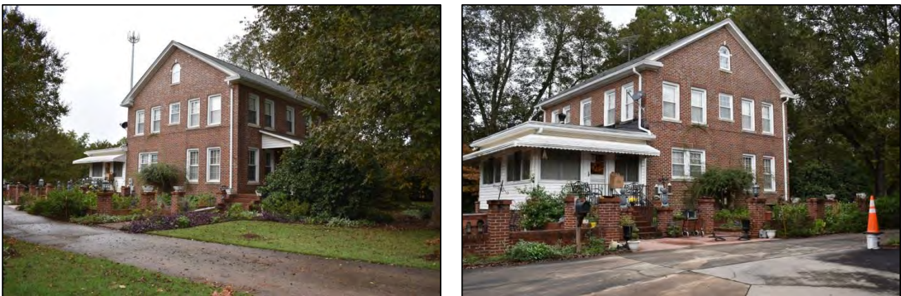
Figure 20: Left, view of northeast corner of the ZumBrunnen House; right, view of side (eastern) and rear elevations.
