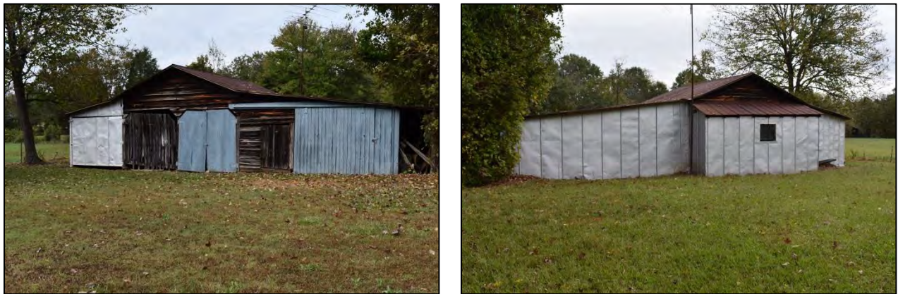
Figure 7: Left, view of eastern elevation; right, view of western elevation.
