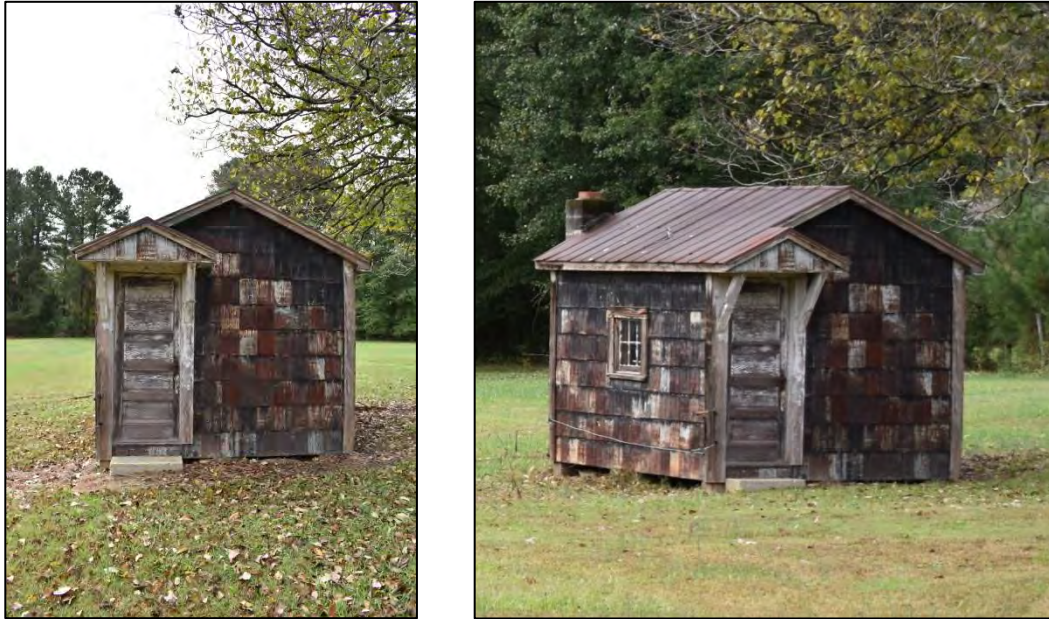
Figure 8: Left, view of front (northern) elevation; right; view of northeast corner.
