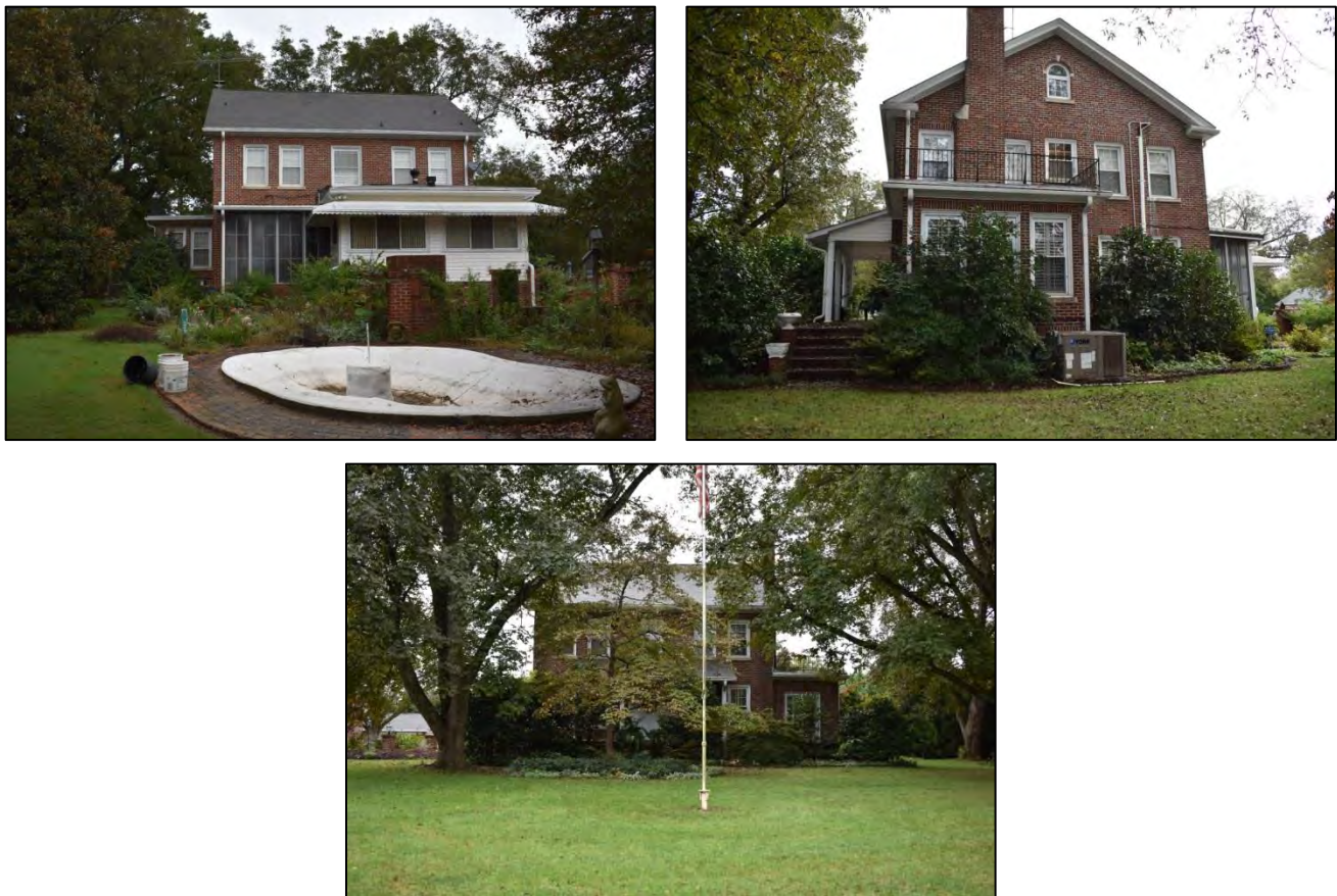
Figure 21: Left, rear (southern) elevation of house; right, view of side (western) elevation; center, front (northern) elevation.
